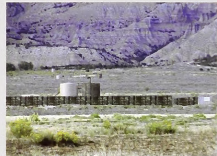
A stand-alone fiberglass screen blocks the view of a well pad. The pattern can be customized to better match the landscape. Photo credit: www.LBIE.com
